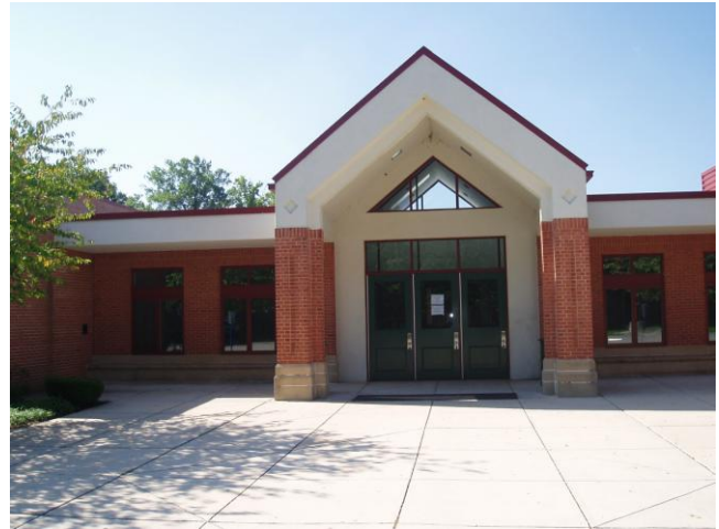
Gum Springs Community Center
