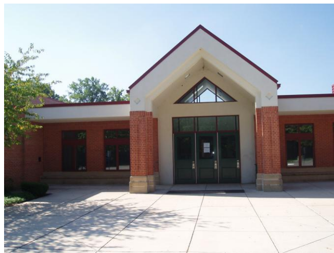
Gum Springs Community Center
