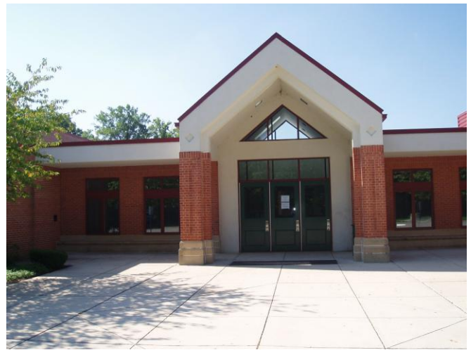
Gum Springs Community Center
