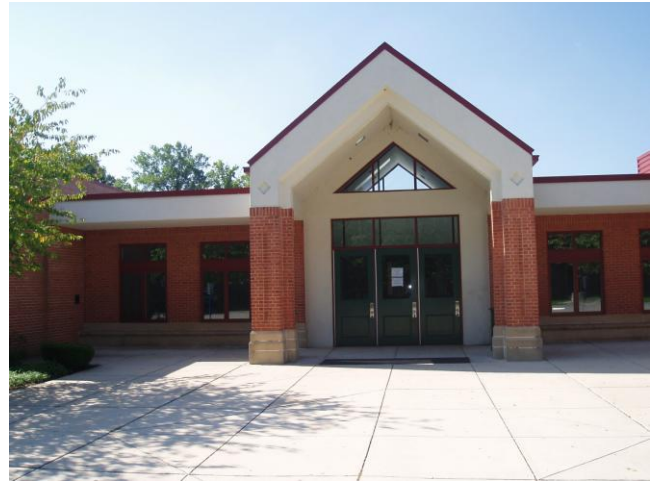
Gum Springs Community Center
