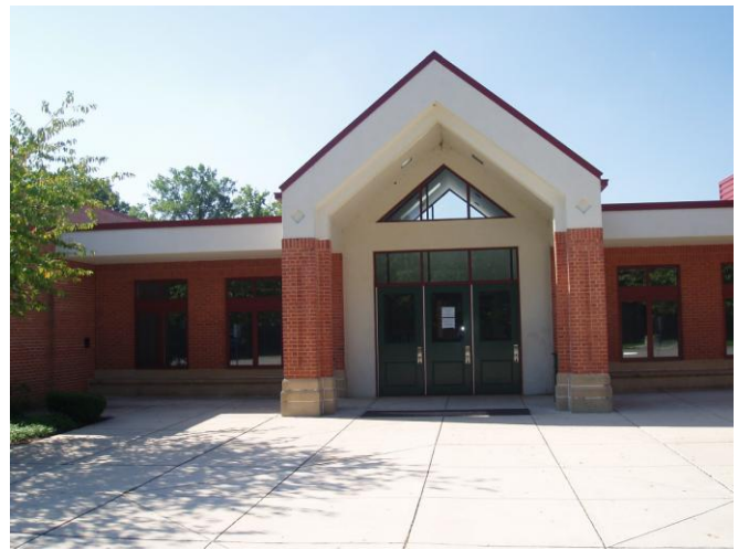
Gum Springs Community Center
