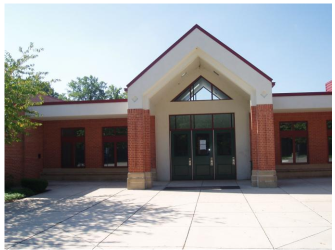
Gum Springs Community Center
