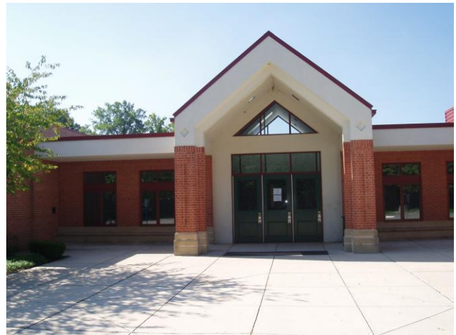
Gum Springs Community Center
